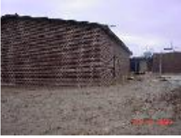
Safe Room on Harrisburg campus 2004
