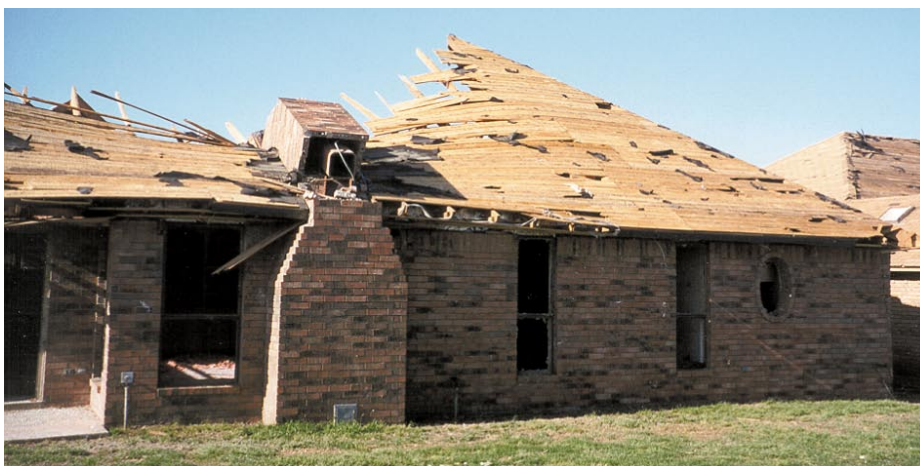
Avoid selecting a refuge area that is near a masonry chimney (Moore, OK).
