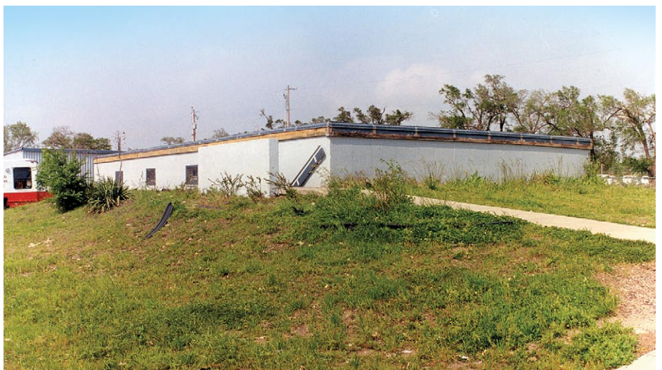
View of a partially below-grade community shelter at a manufactured home community (Wichita, KS).
