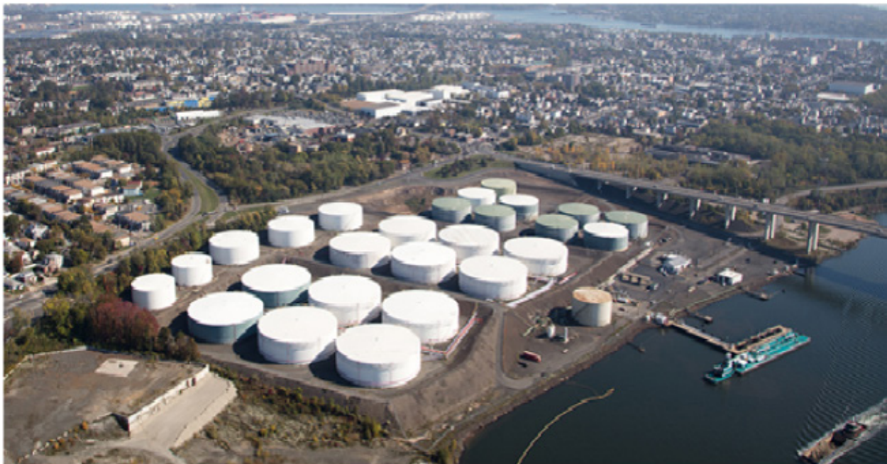
Figure 2: Storage Tanks Holding Northeast Gasoline Supply Reserve and Commercial Supplies at Raritan Bay Facility in New Jersey
