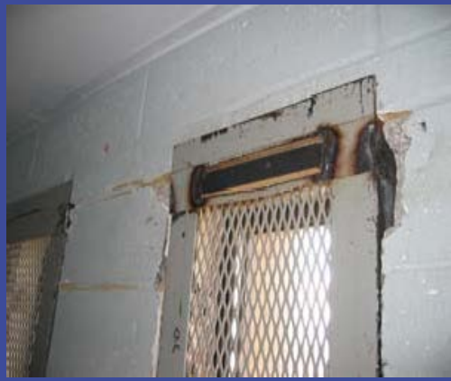
Loosely encased wire meshed windows at a detention center.
