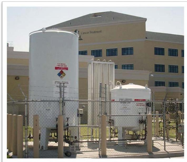
Figure 1. Liquid Oxygen Storage Tanks, Image Courtesy of Chart Industries
