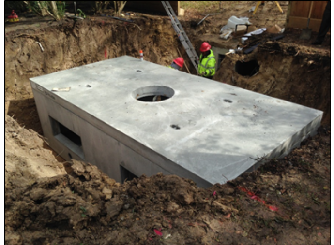
Drainage boxes in Bunker Hill were installed throughout the neighborhood for flood prevention. Photo courtesy of Karen Glynn.
