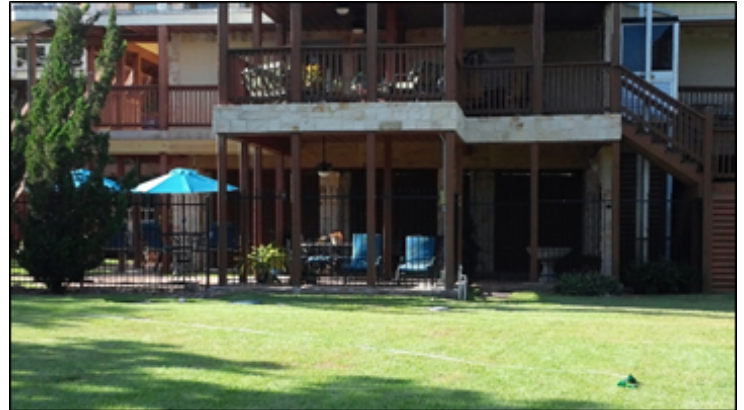
Figure 2 - A parking space and patio were created underneath the home because of the elevation project. Photo by Mary Sullivan
