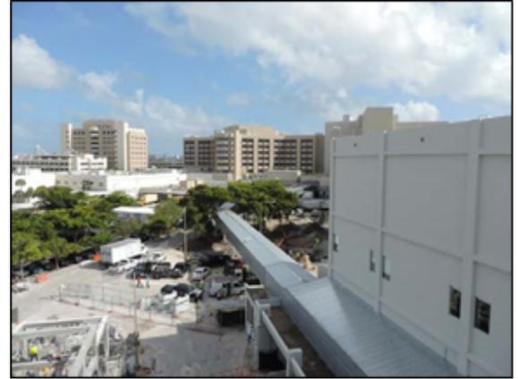
Supported by steel columns, the hardened utility bridge connects Energy Center Building #1 to the Medical Center. ***Photo courtesy of Florida Division of Emergency Management***
