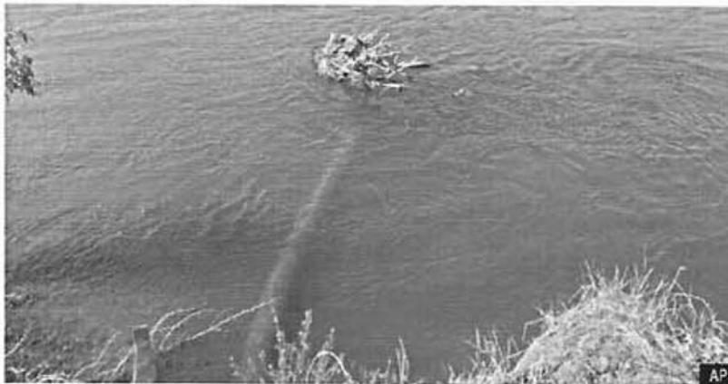
*Exposed pipeline in the river at risk of being ruptured.*
