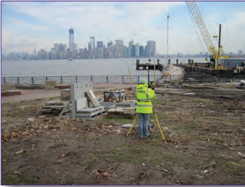
U.S. Geological Survey hydrologic technician surveying a high-water mark on Liberty Island, New York, following Hurricane Sandy.
