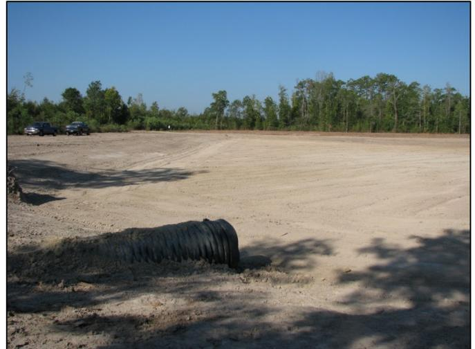
**Pipe in foreground is the part of the flood control mechanism that lets flood waters out of the pond once the flooding event is diminishing. A spillway located between pond and Tiger Creek allows flood waters to enter pond.**
