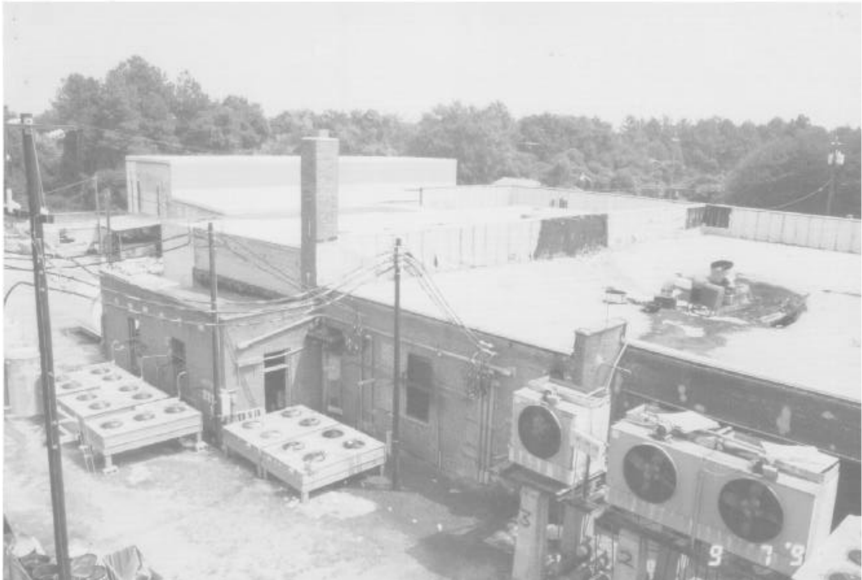
A view from the aerial ladder from the west side looking to the northeast. The roof collapse can be seen on the right, refrigeration compressor equipment is seen on the ground in the lower left.
