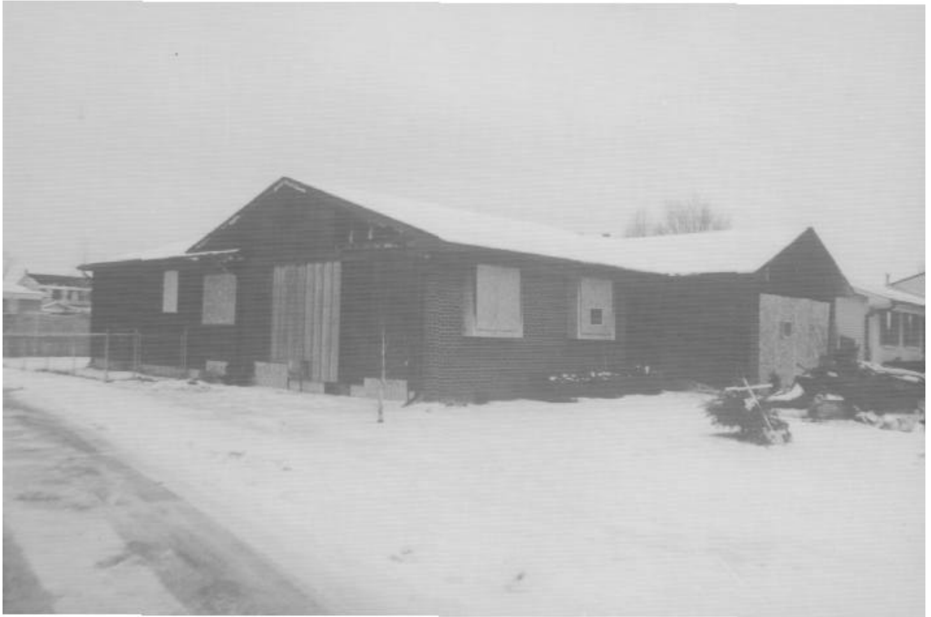
Front view of the home and exposure side two.
