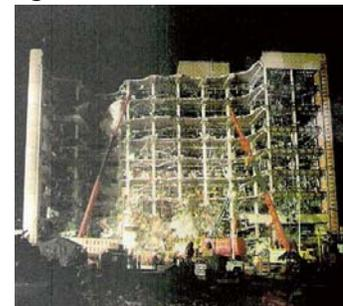
*Temporary power lines and poles, floodlights, and light towers supplied power and light for nighttime operations.*
