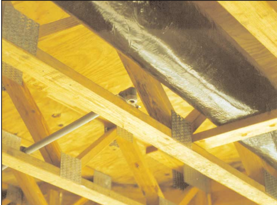
12. The parallel cord wood floor trusses used in the original construction and a polybutylene automatic sprinkler line.
