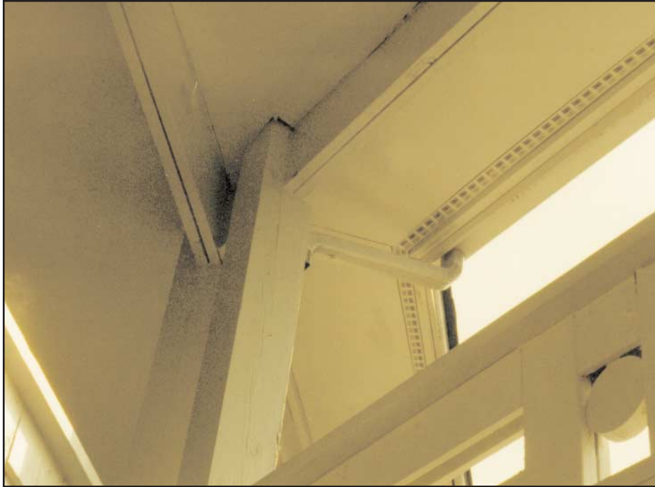
11. Typical eave line vents installed around the perimeter of the building. The fire is believed to have entered the attic through these vents.
