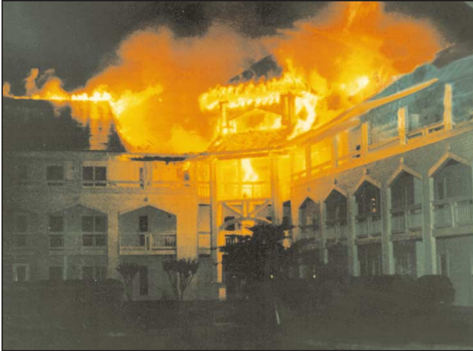
5. Fire involvement in Sector D (North side) as units were preparing to operate in this sector. The fire was well-established in the attic, third floor walkway, and fourth floor.
