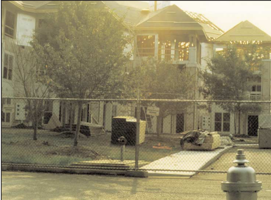
6. Fire hydrant and core siamese connection used by Engine 54 on arrival. Repairs and reconstruction are being made to the front wing; this side is the patio/balcony for each apartment.
