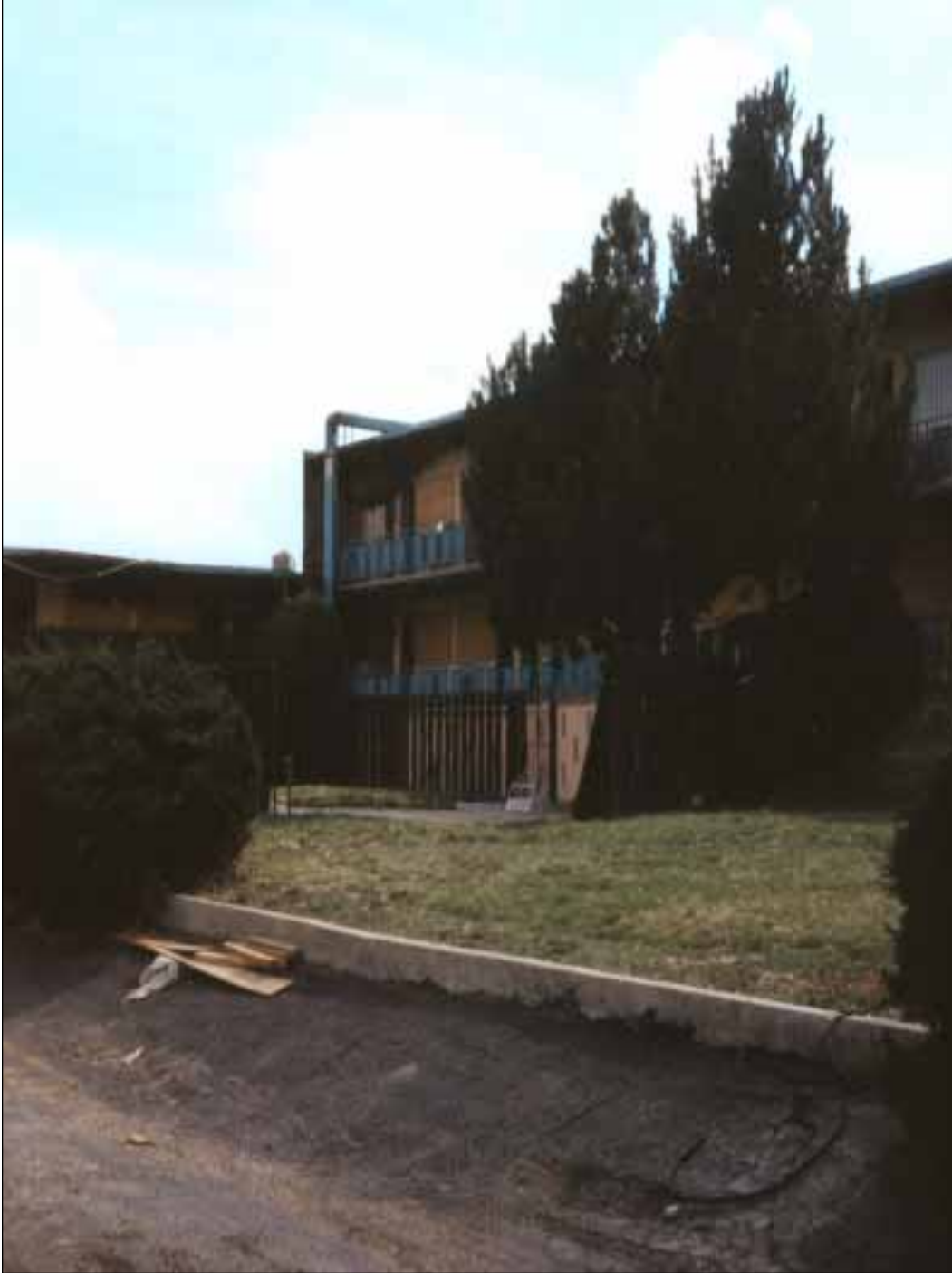
3. The inside corner of the junction between the front and west wings; part of the U shape. This illustrates all three levels of the property and the grade change.
