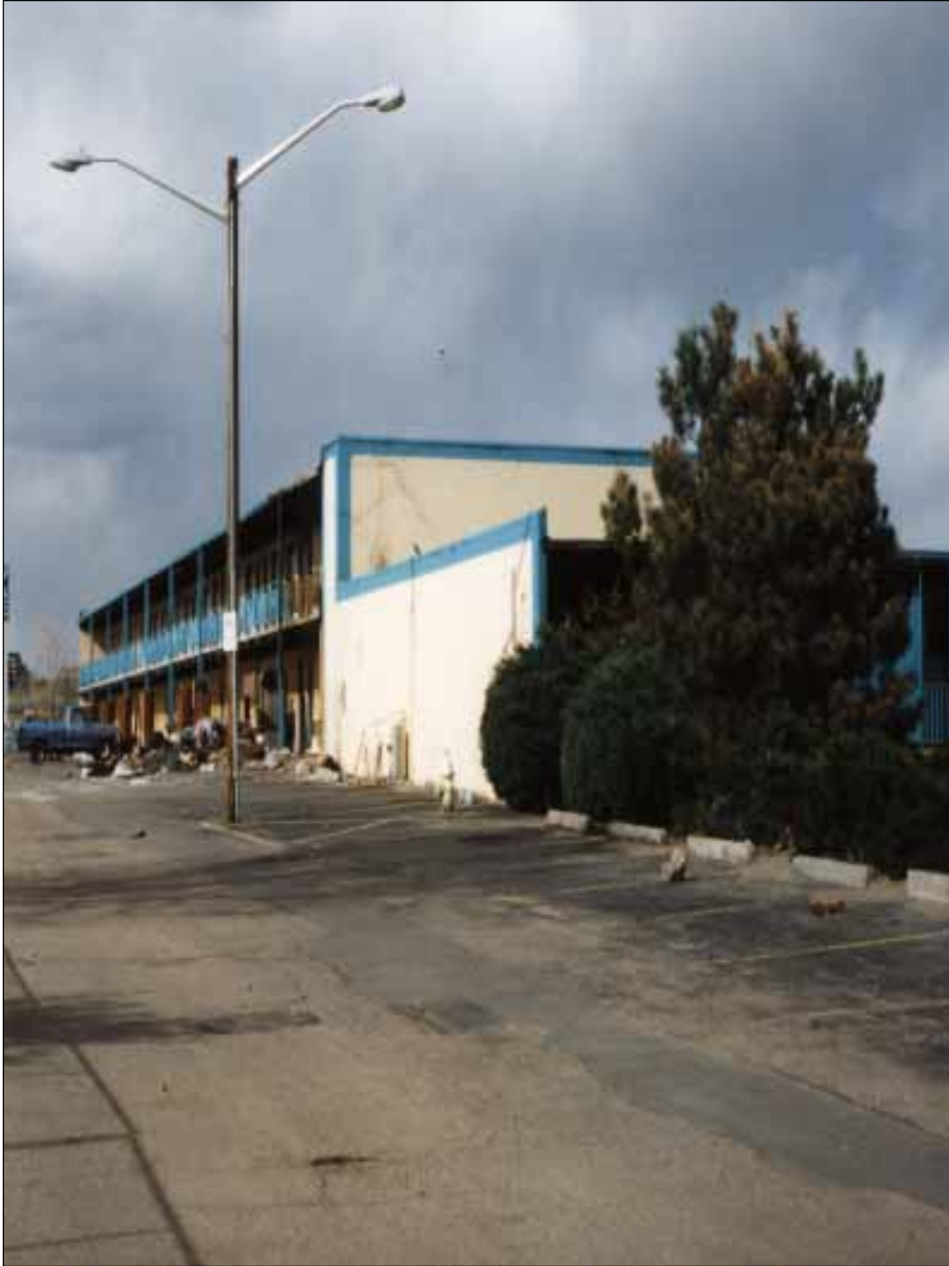
2. The west side of the property looking north. This is the 200 and 300 level guest rooms of the west wing and the end of the front wing. Engine 67 used the fire hydrant to the right of the light pole.
