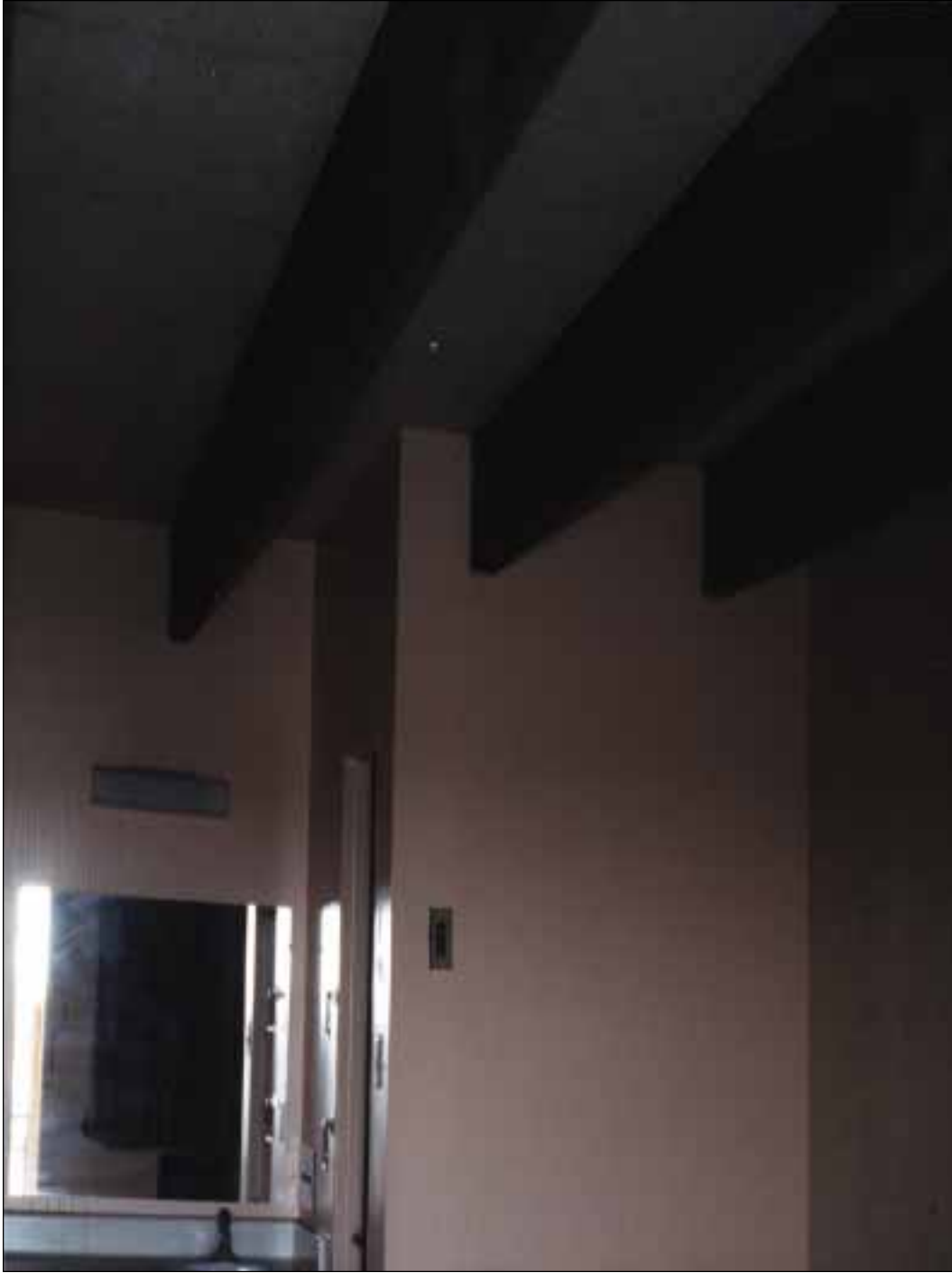
4. Typical guest room ceiling, bathroom, and sink on the utility chase wall.
