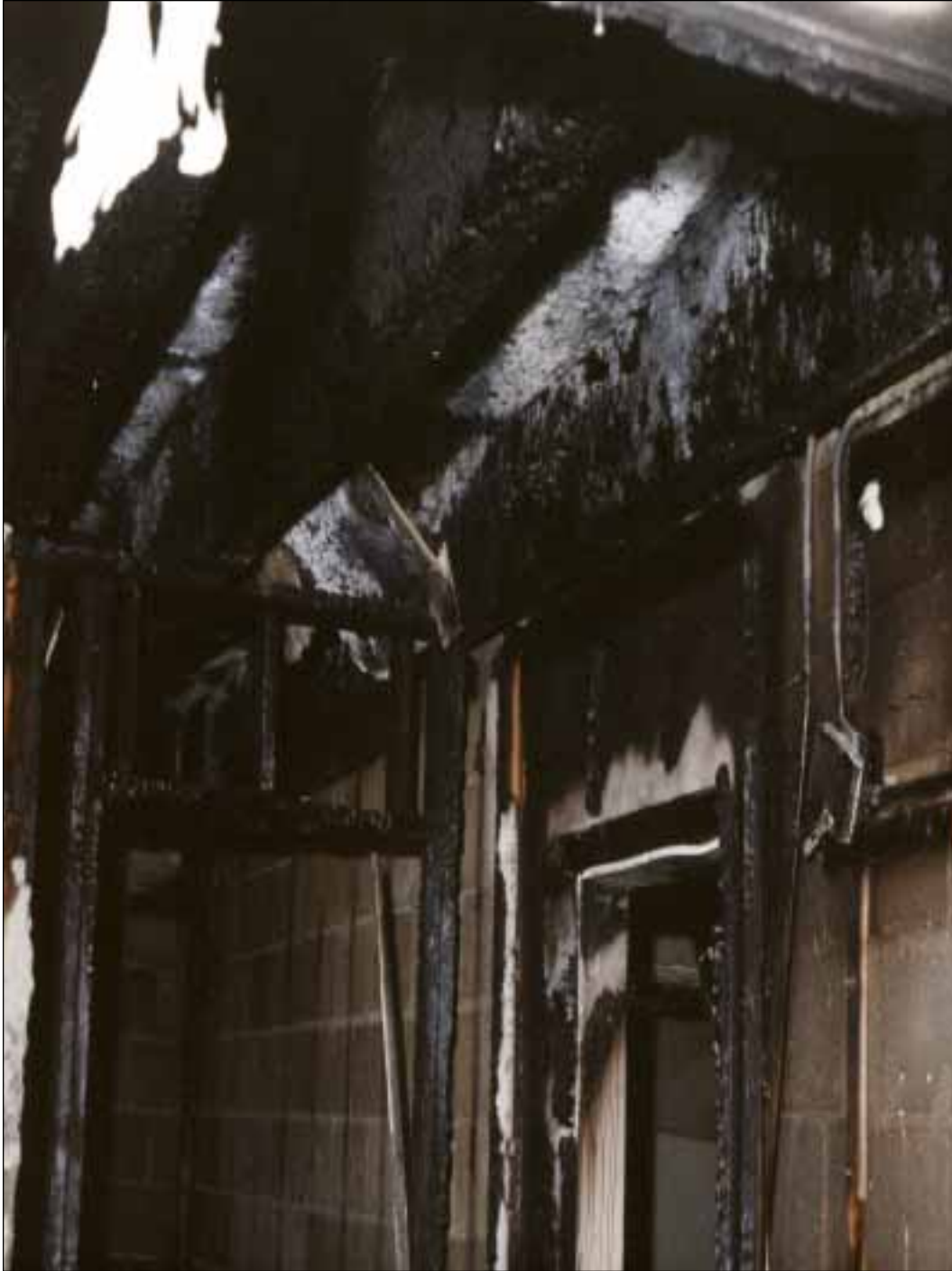
10. The top of the door frame for the 100 level closet determined to be the point of origin. The open stairway to the 200 level is to the top left off the photograph.
