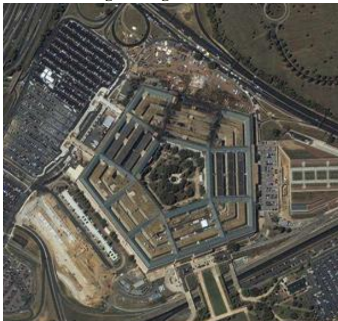
Figure 4. Aerial View of Pentagon Showing Damage
