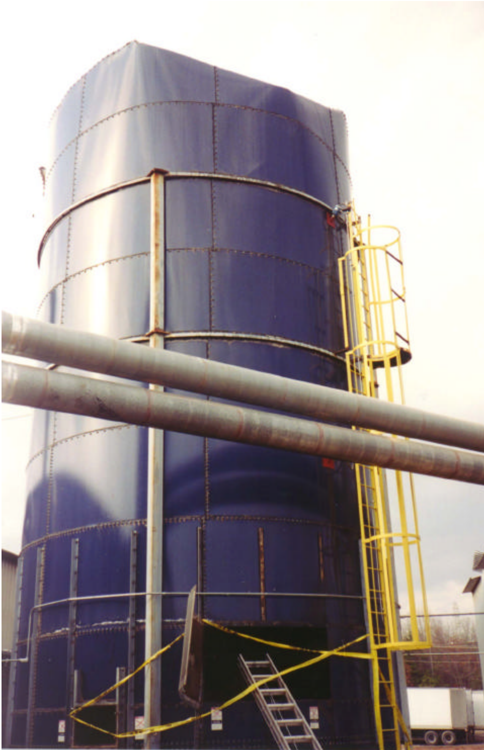
Photo 2. Access plate, origin of explosion
