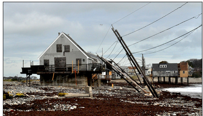
House damaged by Hurricane Sandy (Source: FEMA)
