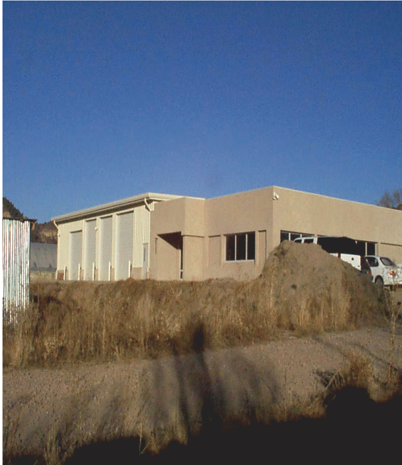
Facility in Dulce, New Mexico, used to construct new engines, that was completed in FY 1999 with fire deferred maintenance and construction funding
