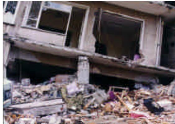
**Figure 1: Partially Collapsed Building from Turkey Earthquake**
