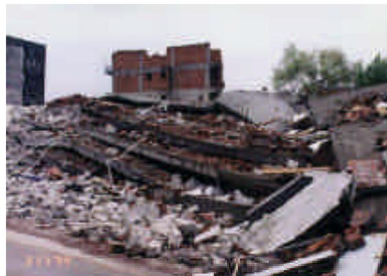
**Figure 2: Totally Collapsed Building from Turkey Earthquake**
