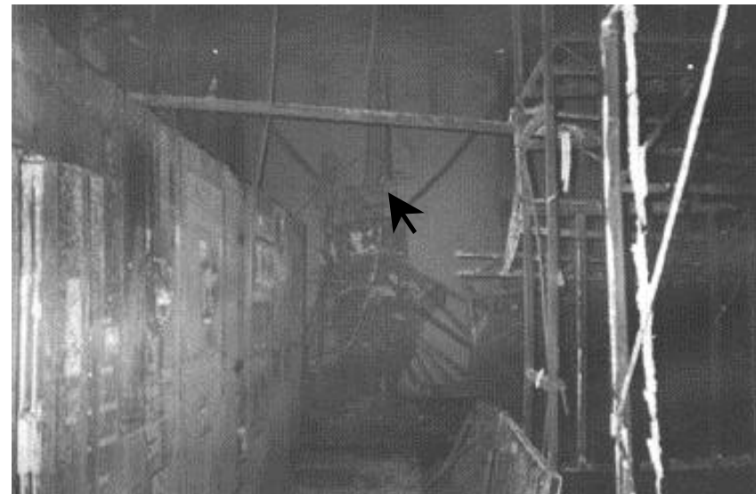
Remains of some scenery prop frames which were obstructions to hose line advancement and locating the fire. Also visible hanging from the ceiling is the wire mesh used to support the spray-on fire protection which was damaged during the floor renovation.
