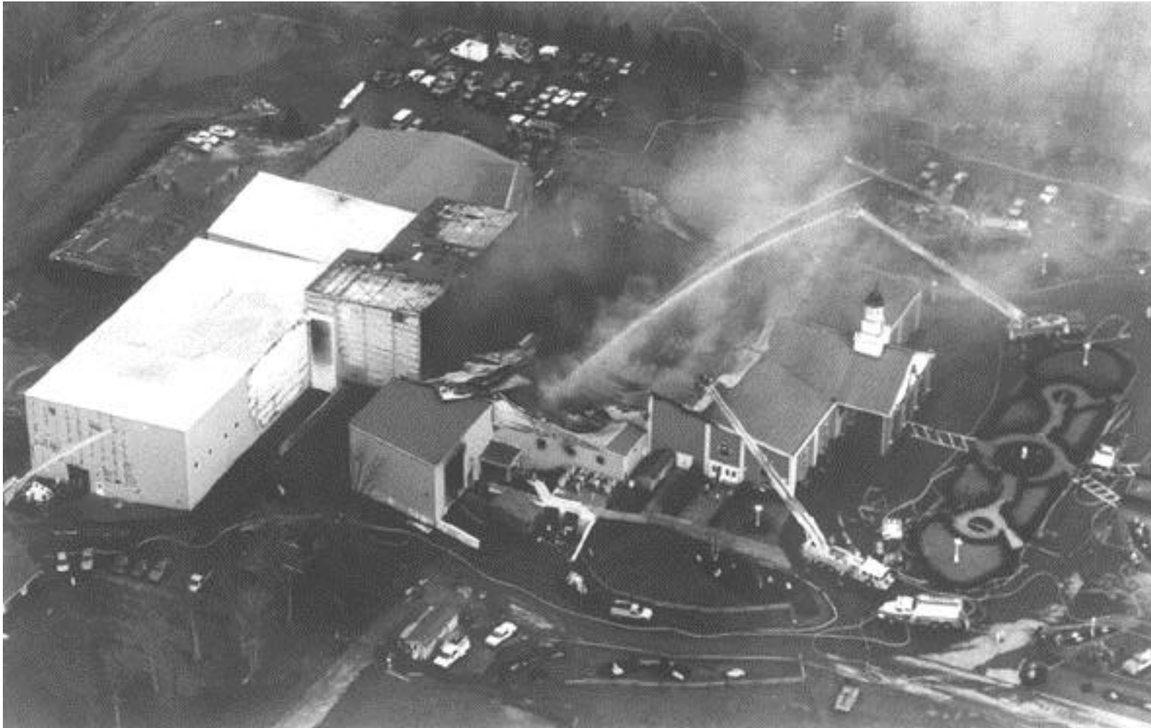
Aerial View One – shows the fire in progress after the auditorium roof collapsed. Note the four master streams and tanker relay hose lines.
