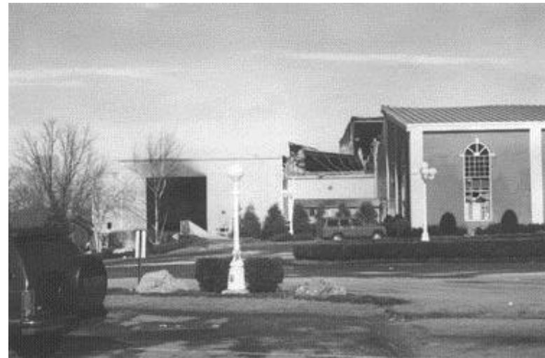
This picture is taken from the front, looking toward side two of the building, which shows the auditorium roof and side stage roof collapse.
