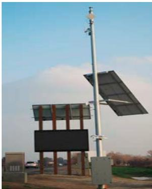
**Figure 1. Typical sensor array for CA's fog detection and warning system**
