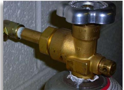
Control valves for compressed gas cylinders are manufactured with various internal or external thread connectors to ensure that they are compatible with the gases stored in the cylinder.
