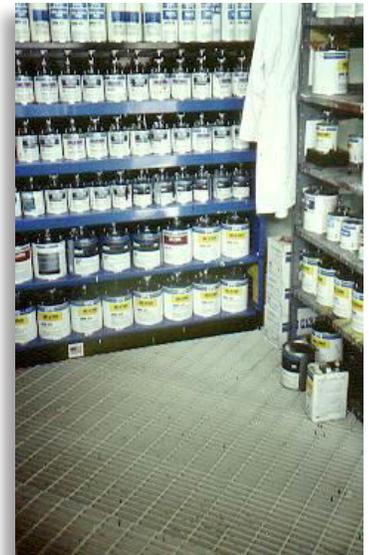
This flammable liquid storage room combines spill control and secondary containment into a single sump located below the grated floor deck.
