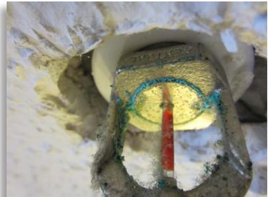
The corrosion around the cap of this recalled Central ELO-LH wet sprinkler increases the likelihood that it will not operate when needed. (Photo/Byron Blake)
