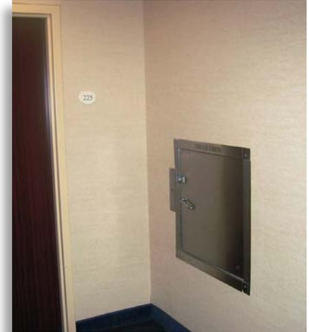
Refuse and linen chutes must be constructed to prevent the spread of fire products, including fire-resistive opening protectives, as illustrated here from an older version of a building code. Openings into corridors are not permitted in current codes.
