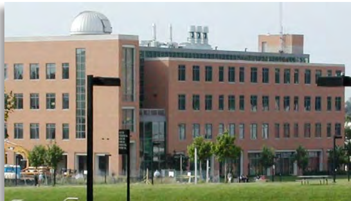
A building like this – with multiple stories and varied hazardous operations – may have more than one sprinkler design area of application.
