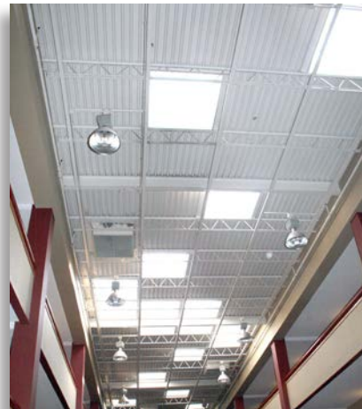
The area of application is the area where it is assumed that all sprinklers will operate simultaneously to control a fire.
