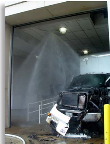
Density in sprinkler design refers to the amount of water per square foot (square meter) that the system is intended to deliver each minute. (Photo/Keith Heckler, Rockville Fire Department, Maryland)
