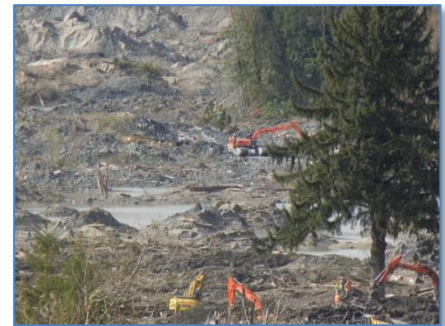
Heavy equipment at the 530 slide site April 10. – Bronlea Mishler
