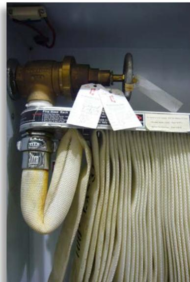
The water accumulated in the first hose bend downstream of the hose station is a sign that this Class II standpipe hose should be checked for damage.
