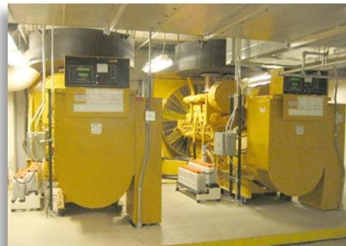
These diesel-powered generators provide an emergency power supply for a high-rise office building.
