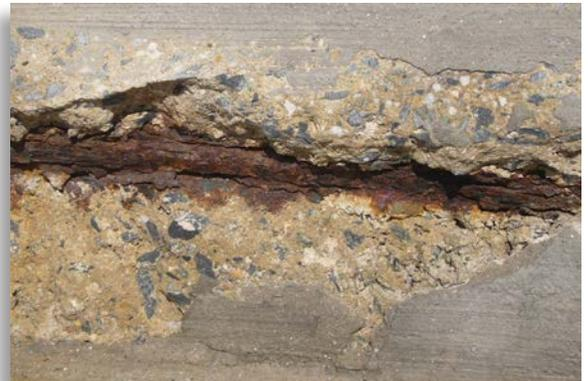
The concrete that once protected this steel reinforcing bar has spalled, exposing the reinforcement to the elements, including the heat from a fire.
