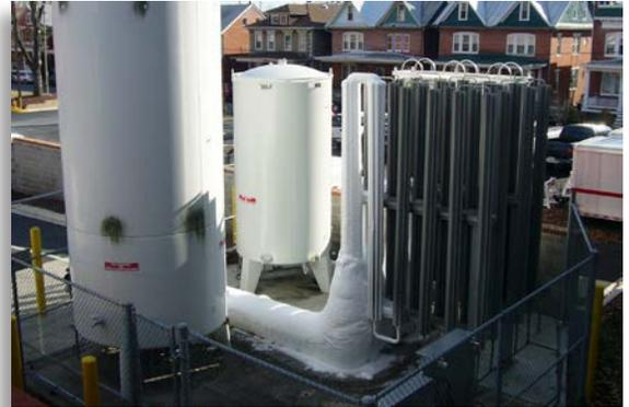
This bulk liquid oxygen container and vaporizer (right) are part of a hospital's medical gas system.
