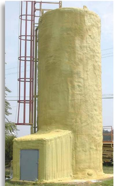
This water tank that supplies an automatic sprinkler system is protected from freezing by a combination of spray-on insulation and immersion heaters.
