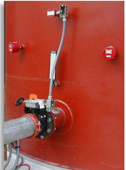
The outlet pipe from this 15,000-gallon (56,780-liter (L)) aboveground water storage tank supplies an automatic sprinkler system.
