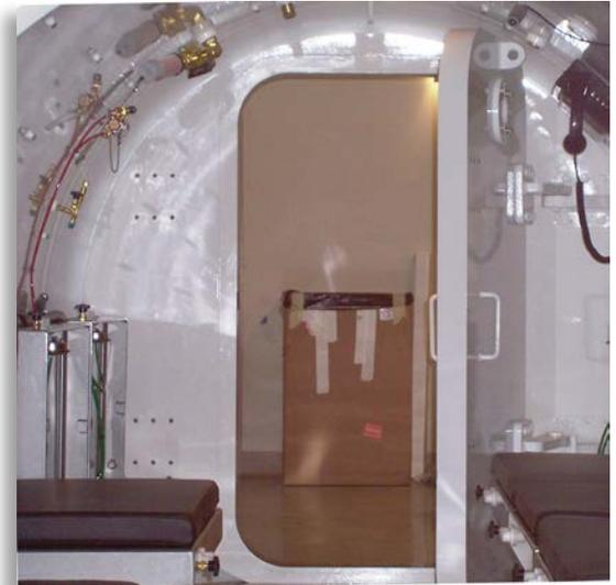
The oxygen-rich environment in this recompression or hyperbaric chamber is protected by a high-pressure, water-mist fire protection system.
