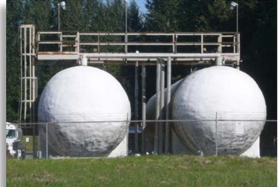
These containers are insulated to help keep the cryogenic carbon dioxide liquid cold.
