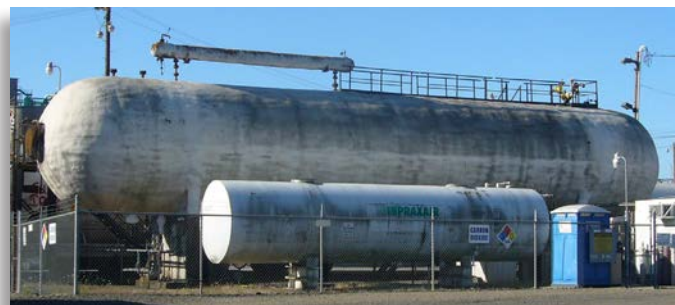
These vessels contain carbon dioxide, a gas that is commonly stored as a cryogenic fluid.
