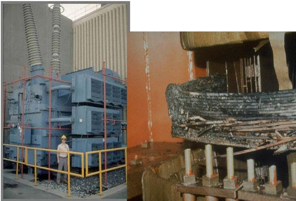
Figure 2. Step-up transformer damaged at Salem Nuclear Generating Plant due to geomagnetic storm on March 13, 1989. Images provided by Public Service Electric and Gas and taken by Peter Balma (pictured). Photograph on the left shows the outside of the damaged transformer for scale. Photograph on the right shows some of the physical damage to the internal components of the transformer.
