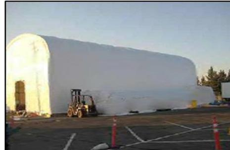
Figure 1. Two story building, without and with secondary containment (tenting), at Idaho National Laboratory.
