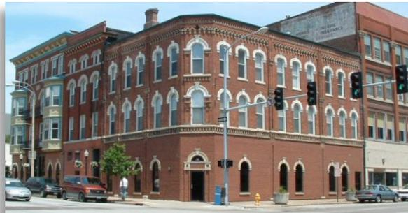
Using this three-story, nonsprinklered masonry office building as an example, this structure has an Insurance Services Office (ISO) needed flow of 750 gallons per minute (gpm).
