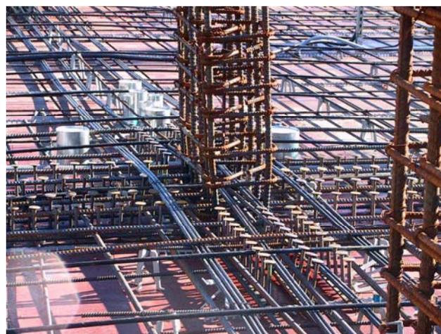
Shear stud reinforcement in slab-column connection. Photo courtesy of Eduardo Miranda.
