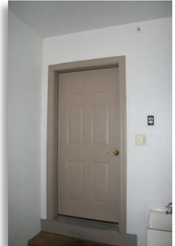
The photo shows the installation of a single sprinkler head on the interior wall adjacent to the entry door from the garage to the home. (The head can be seen to the top right of the door.)
