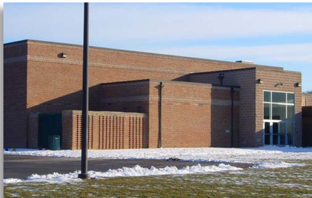
This one-story, noncombustible building will have a “construction factor” coefficient of 0.8 in the Insurance Services Office (ISO) “effective area” subformula.
