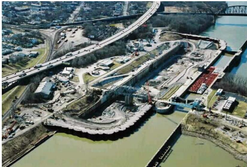
Figure 6: Construction of second 1200-foot lock chamber at McAlpine, July 2004. The existing 1200-foot lock at right is being closed for gate repairs, halting all through traffic.
