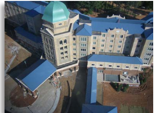
This metal roof covering may achieve a Class A, B or C fire resistance rating depending upon how the structure beneath is protected from fire. Photo courtesy of Wayne Powell.
