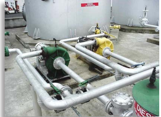
This product transfer piping must be installed and tested so it is liquid tight.
