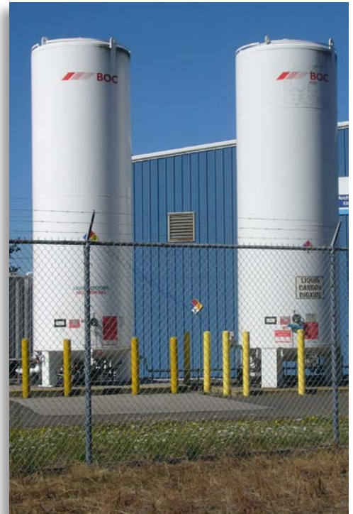
The quantity and environment for hazardous materials can be regulated through the use of fire code permits.
